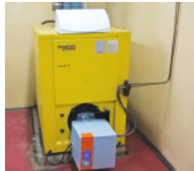
Photo 32. Old oil-fired boiler in one of the pilot buildings
