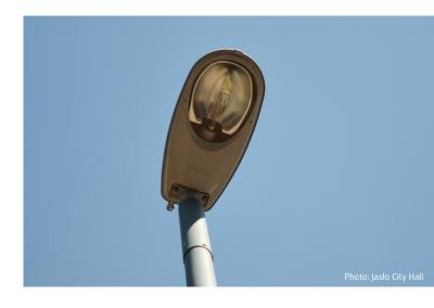
as the power limiters. Thanks to the latter new lamps consume less electricity when the road traffic is lower. Old luminaires - mostly mercury lamps - had large capacity (over 250 W), were outworn and often failed. New sodium luminaires have considerably lower capacity: 70, 100 and 150 W. For the long time they will not need intervention from the repair services, which will also significantly reduce maintenance costs.
